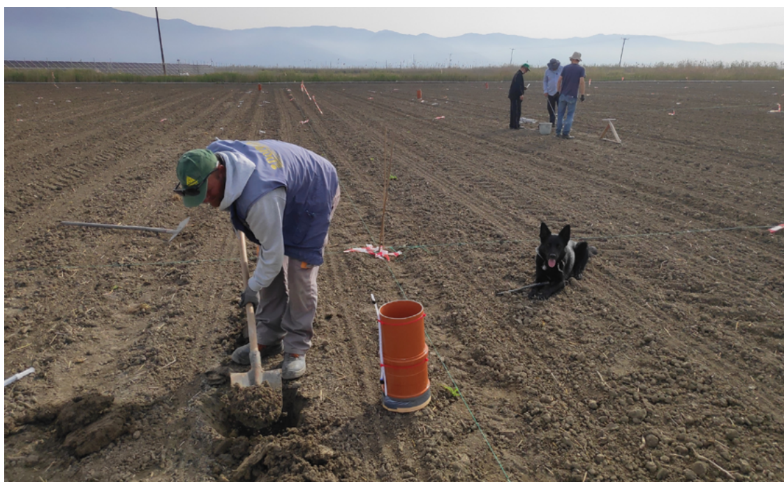
Figure 6.47. Doris digging out a hole to install the orange lysimeter to the right of him. Due to the size of the lysimeters, they only just fit in between two rows of cotton seeds (note the parallel marks from the cotton sowing that run all across the field) and he needs to be careful to minimise disturbance of the cotton seeds. In the top right corner Lefteris and his colleagues from the Institute are installing macrorhizons in experimental plots.
